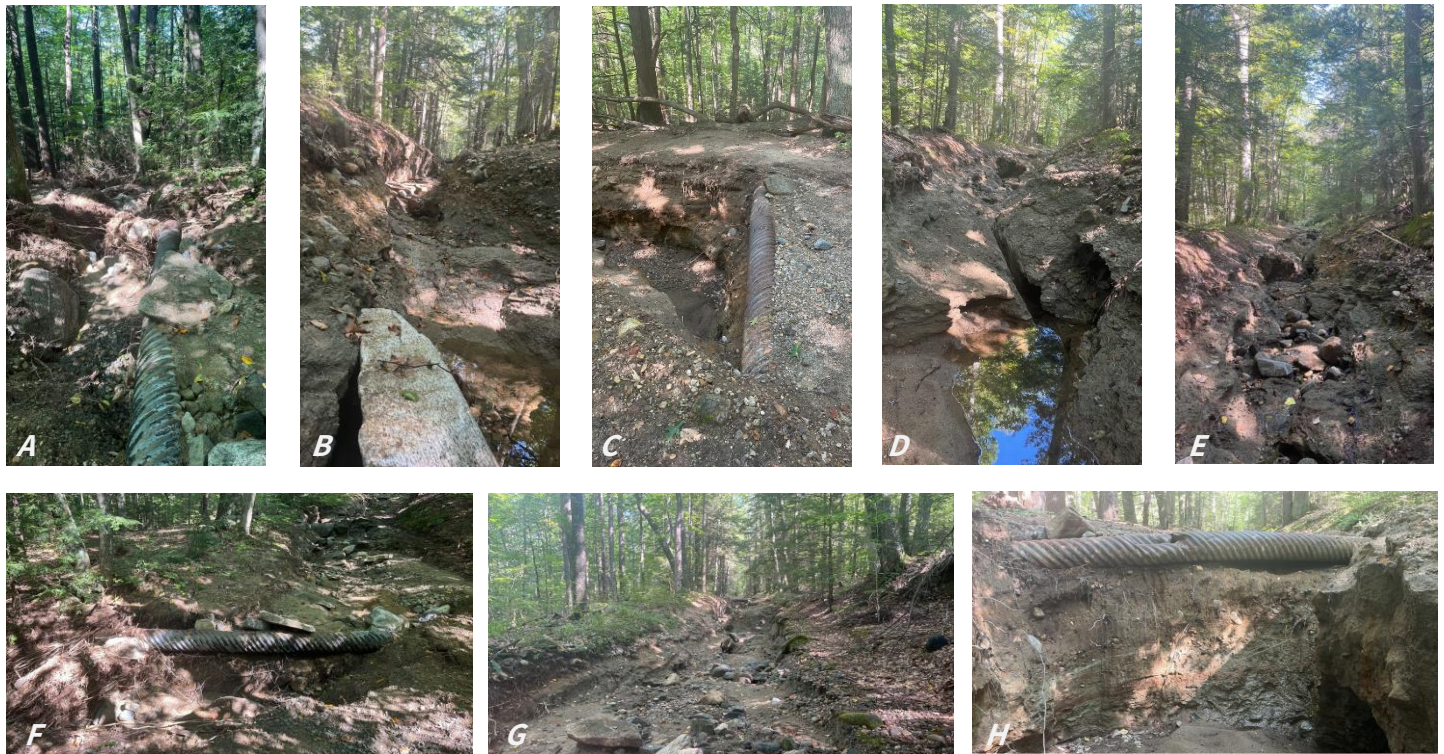
A & F: A culvert at the fork in Talbot Hill Rd has been uncovered due to July 2023 storm erosion and serves as a barrier, sending stormwater down a stream channel that carved a ravine. B, D, E & G: Damage from the storm destroyed Talbot Hill Rd. C & H: The July 2023 storm caused erosion up to six feet deep. The entire soil profile is visible at the second culvert.
