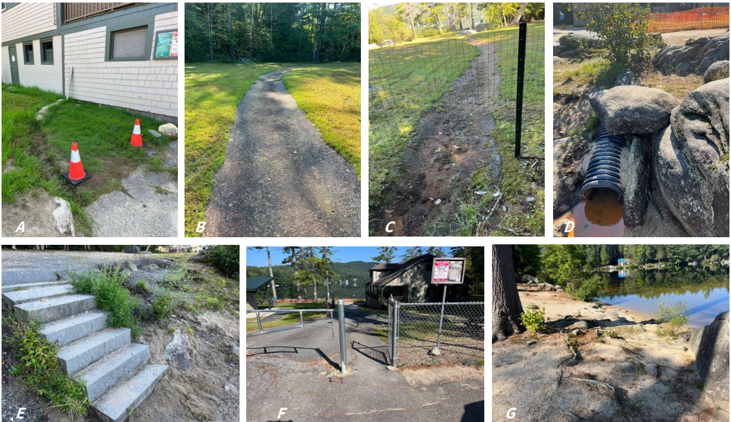
A: Erosion channel leading under the building towards a drain inlet. B and C: Paved swales funnel stormwater to a single discharge point. D: Overflow from a rain garden discharges to the lake via a plastic pipe. E: Granite steps leading to the water's edge. F: Highly impervious parking lot ultimately drains to the lake. G: Shoreline erosion from an area of bare soil combined with an inadequate shoreline buffer.
