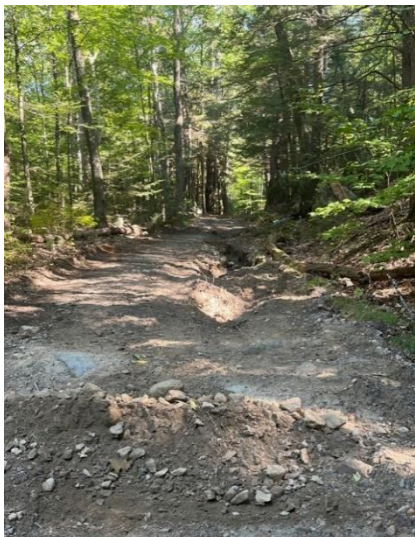
(Left) Erosion gullies down the bottom of Talbot Hill Rd at Site 3-07. (Right) Multiple gullies were observed over the entire length of Site 3-07.
