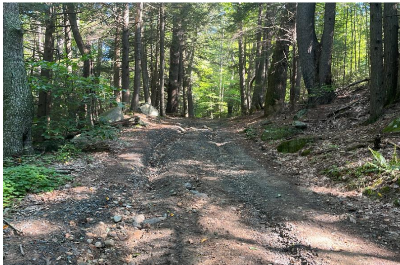
(Left) Erosion gullies down the bottom of Talbot Hill Rd at Site 3-07. (Right) Multiple gullies were observed over the entire length of Site 3-07.
