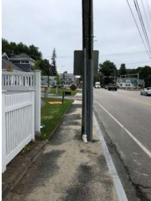
Figure 34 – Telephone pole obstructs sidewalk along US 202 S
