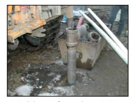
Boring holes to test for ground contamination
