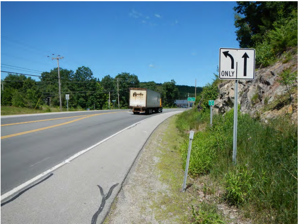
Swanzey, Flat Roof Mill Road-Northbound at the intersection with Flat Roof Mill Road, left turn lane is short with reduced time to slow down and can cause the driver to overshoot the turn onto Flat Roof Mill Road.
