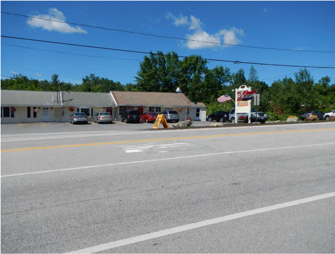
Fitzwilliam: Near intersection of NH12/NH119. Pavement markings are fading; large curb cut into businesses. Signs can cause a distraction to drivers. Sandwich board sign is a sightline hazard for drivers leaving the businesses.
