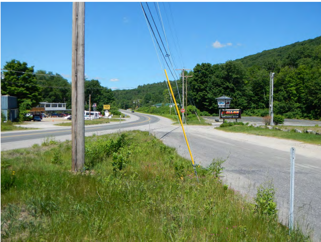
Marlborough, Webb Depot Road- Y- intersection. Consider realigning to a T-intersection.
