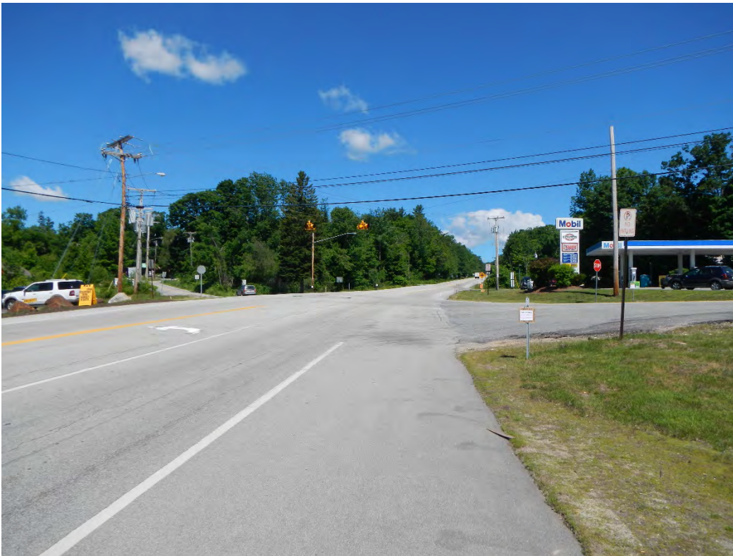
Fitzwilliam: Northbound approach to NH 119 intersection- large area of pavement. Difficult for pedestrians to cross safely and quickly to business. Pavement markings and signs could enhance driver ability to understand turning options.
