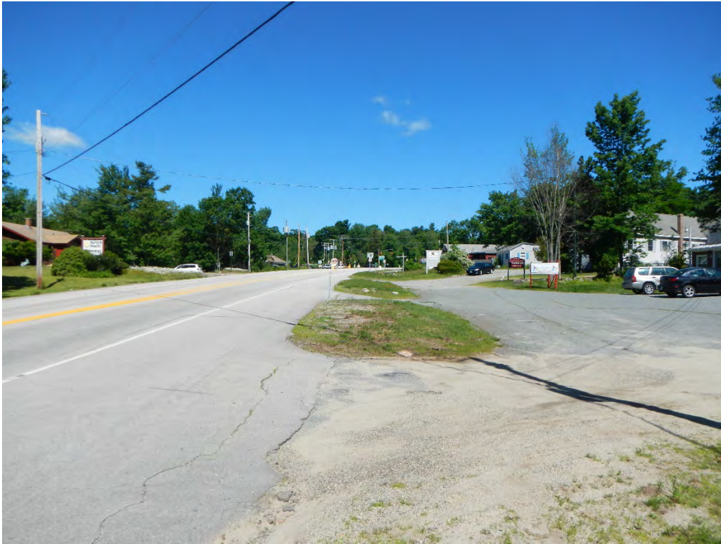
Fitzwilliam: Northbound approach to NH 119 intersection. Access management techniques needed to reduce the points of conflict and reduce driver confusion. There is also a lack of signage and pavement markings to alert drivers of the upcoming intersection.
