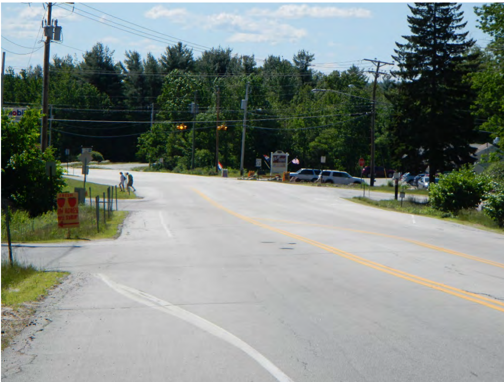
Fitzwilliam: Northbound approach to NH 119 intersection. Access management techniques needed to reduce the points of conflict and reduce driver confusion. There is also a lack of signage and pavement markings to alert drivers of the upcoming intersection.
