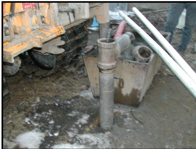
Boring holes to test for ground contamination
